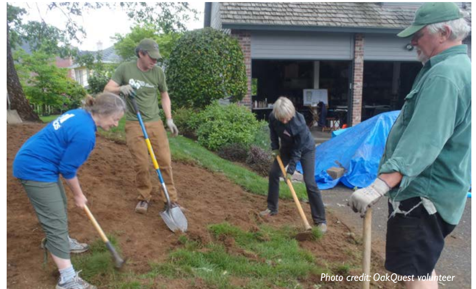
Stripping sod by hand
